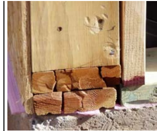
Poor quality timber construction – Split base-plate used.
